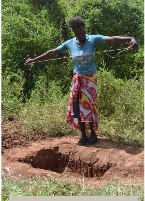
Tendai prepares a hole for the storage of the cattle feed
