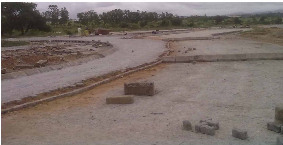
Construction at the “killer junction” along Masvingo Beitbridge road
