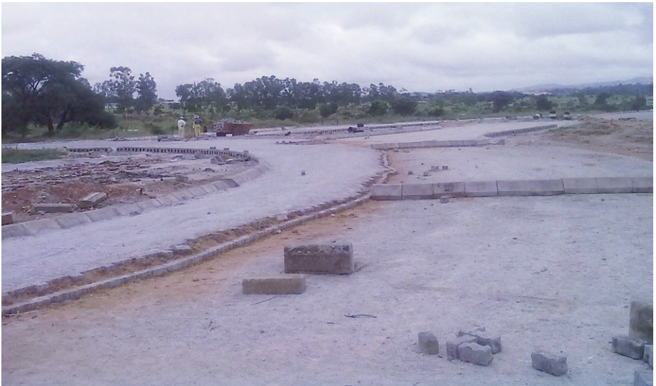
Construction at the "killer junction" along Masvingo Beitbridge road
