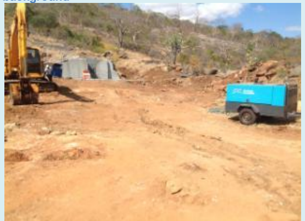
Figure 3: Initial Quarry Site (Mining in Progress)
