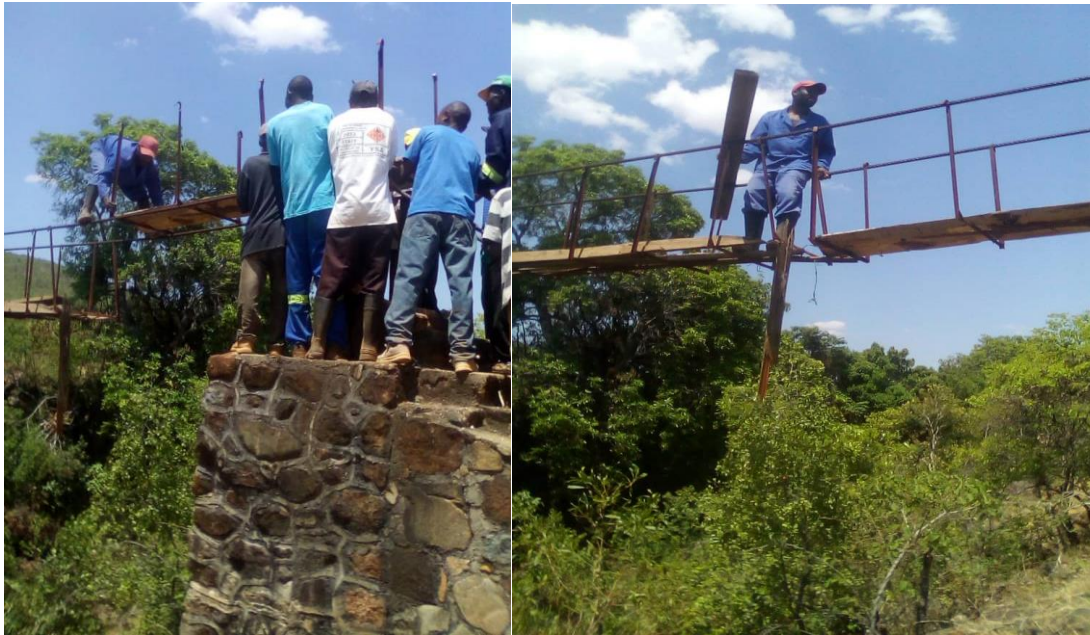
Community members from Manyau Village during bridge construction
