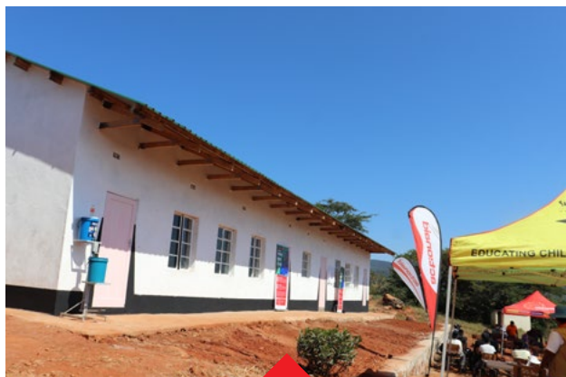
The new classroom block for Tiya Secondary School
