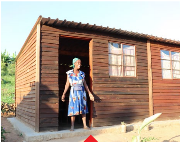
Ever Tekeza from Ward 1 Chimanimani, one of the women supported with temporary shelters after Cyclone Idai destroyed her houses
